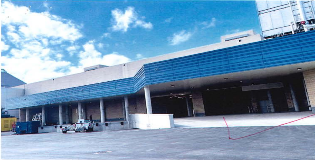
PIC 1 – NORTH LOADING DOCK
