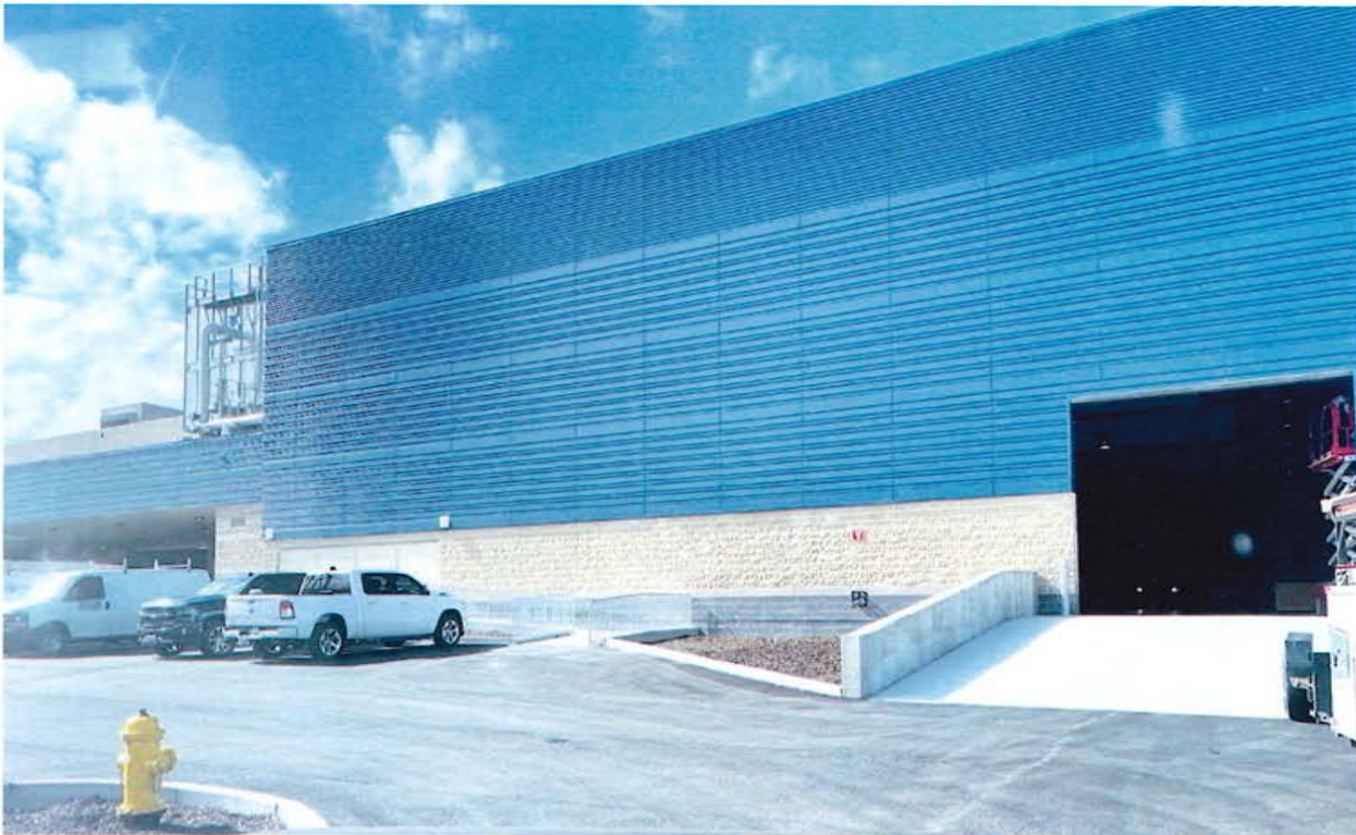
PIC 2 NORTH ROLL UP DOOR – NEW HALL
